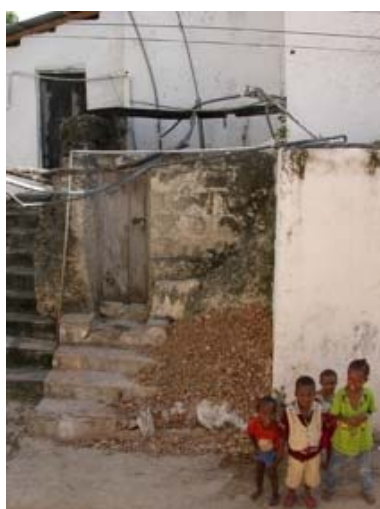
Well and distribution reservoir
