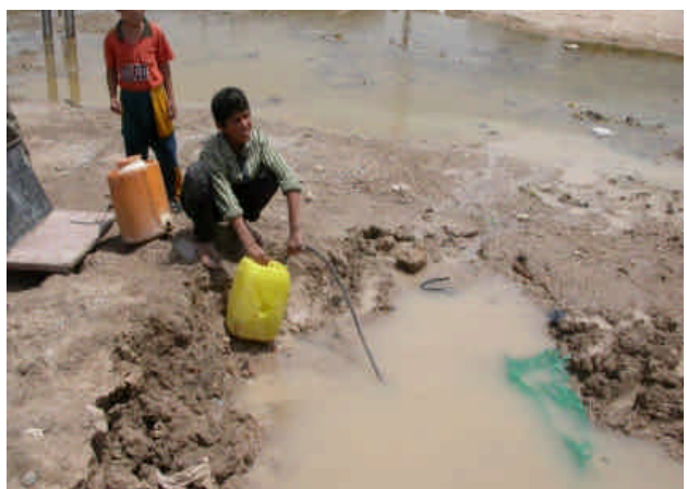
Figure 14 h: Poor tapping in mains
