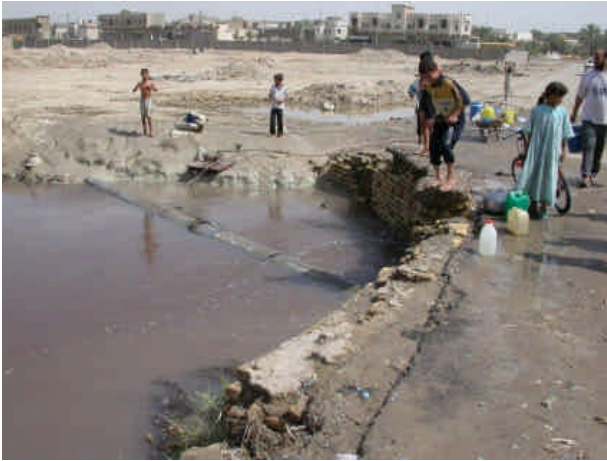
Figure 14 c: Broken AC pipe (General Hospital)
