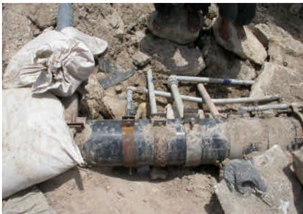
Figure 18 a, b: Illegal branching and connection, to be removed
