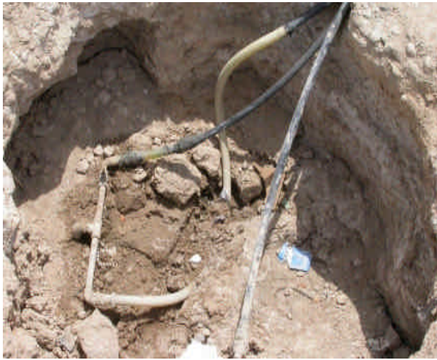
Figure 17 a, b: Makeshift “professional” illegal connection or pump tapping
