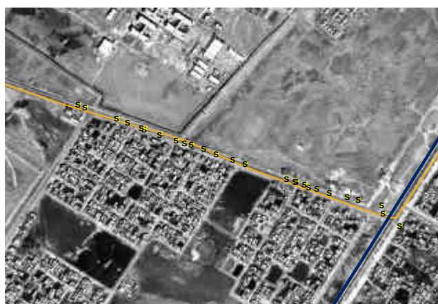
Figure 7: Leaks observed on the raw water pipeline supplying Bradiyah WTS from Wafa al Qaeda. Not yet repaired on 10.05.03.
