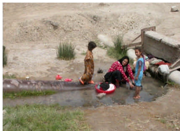
Figure 14 b: Water from leaks on a transmission line
