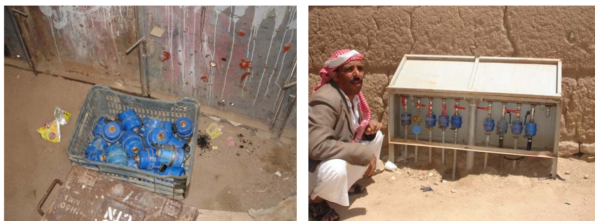
Figure 8 Distribution box and meters ready to be repaired.
