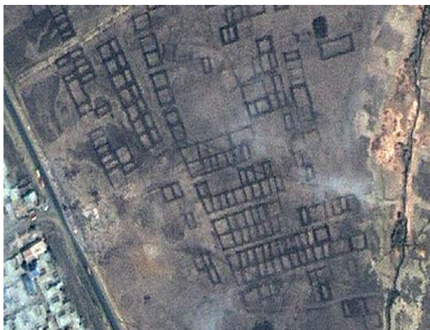
Figure 21 Plots of land ready for construction
