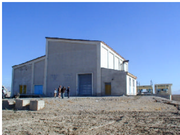
Figure 23 Bagrami High Lift pumping Station
