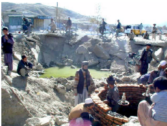
Figures 9 & 10 Damage to the distribution line at the main road leading to Micro-rayon apartment complex and to the 600 mm asbestos/asphalt coated cast iron pipe at the Ghazni road and makeshift repairs (November 2001/P.G Nembrini).
