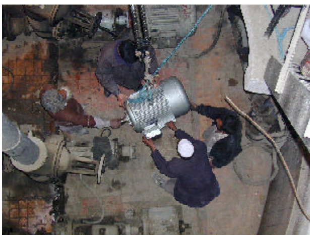
Figure 13 Replacement of the electrical motor of one of the sewage lifting pump in Micro-rayon
