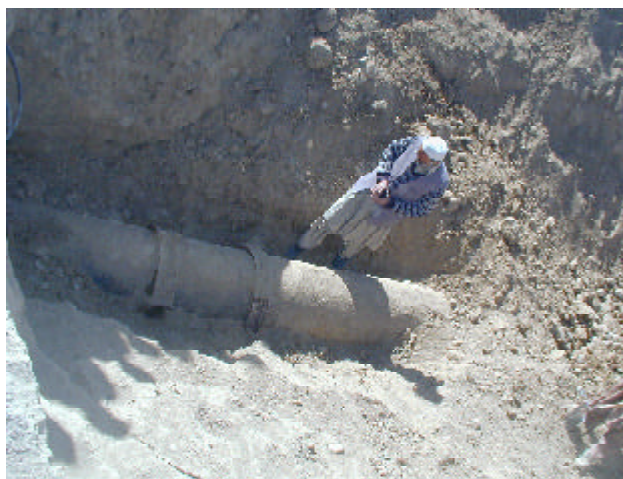
Figures 9 & 10 Damage to the distribution line at the main road leading to Micro-rayon apartment complex and to the 600 mm asbestos/asphalt coated cast iron pipe at the Ghazni road and makeshift repairs (November 2001/P.G Nembrini).
