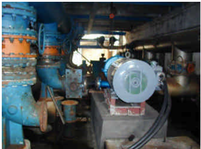
High lift pump with diesel generator and electrical motor
