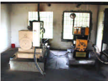
Diesel powered generators
