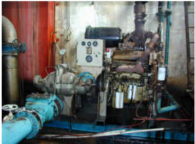
High lift pump with diesel generator and electrical motor
