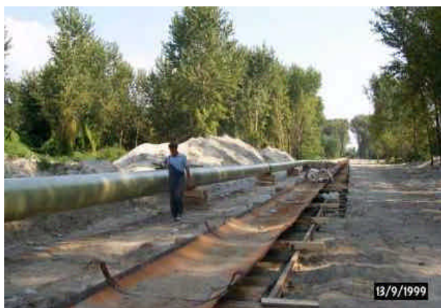
Figure 14 - 16 Dredging the underwater canal and the shores. Preparing the pipeline assembly
