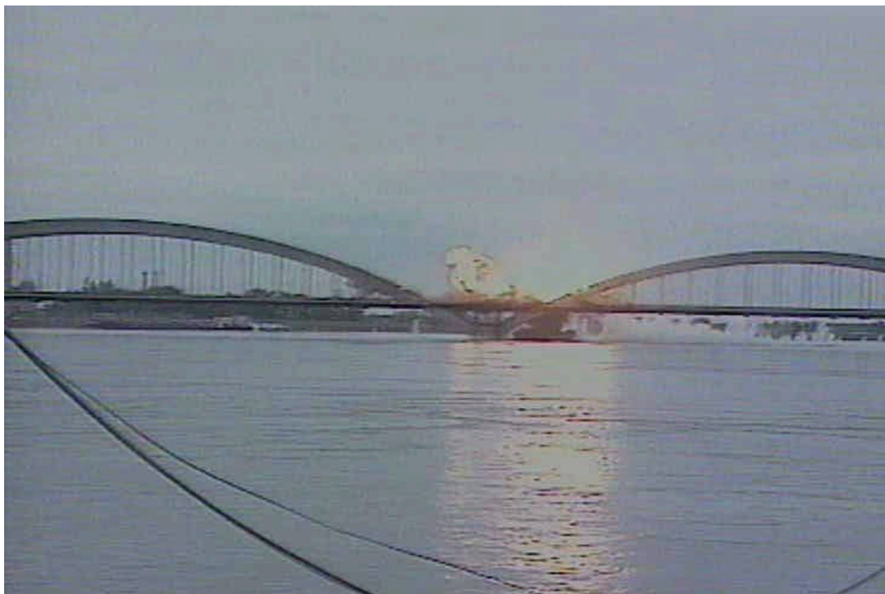
Figure 30 Zezelj Bridge is hit by a missile
