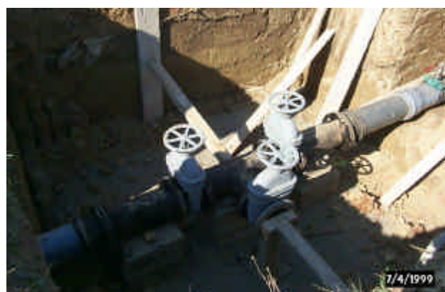
Figure 25 Valves are installed to reconnect the 900mm pipeline to the right bank network
