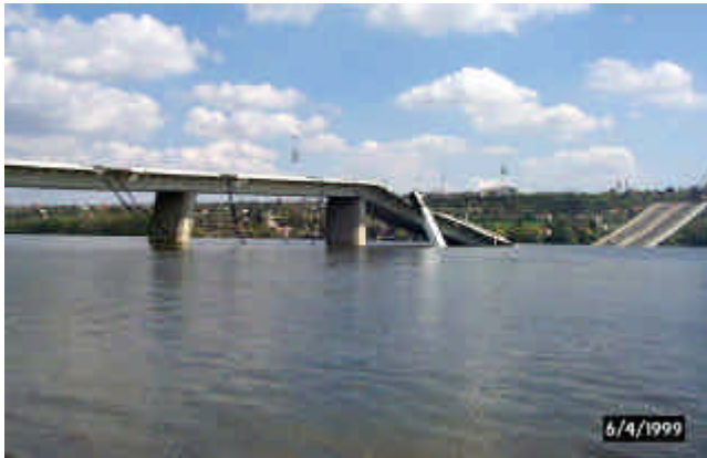
Figure 26 - 27 The damaged Liberty Bridge and drinking water pipelines conveying water over the Danube
