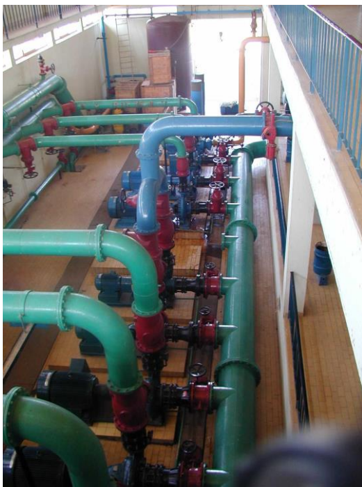
Figure 2 High lift pumps of the new Tshopo treatment station
