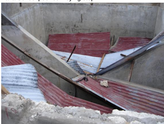
Faza School damaged iron sheet cover of storage tank Ndau Rehabilitation work on the dispensary tank
