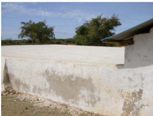
Faza Communal djabia concrete: v.good surface
