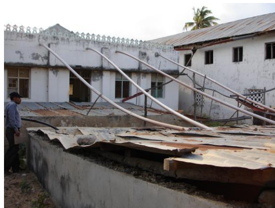
Kisingitini iron sheets oor collection and fair conveying
