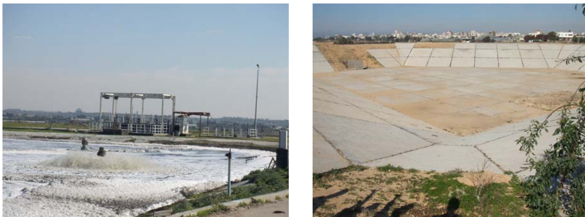
Figure 21: Gaza WWTP under maintenance and with aerators in operation
