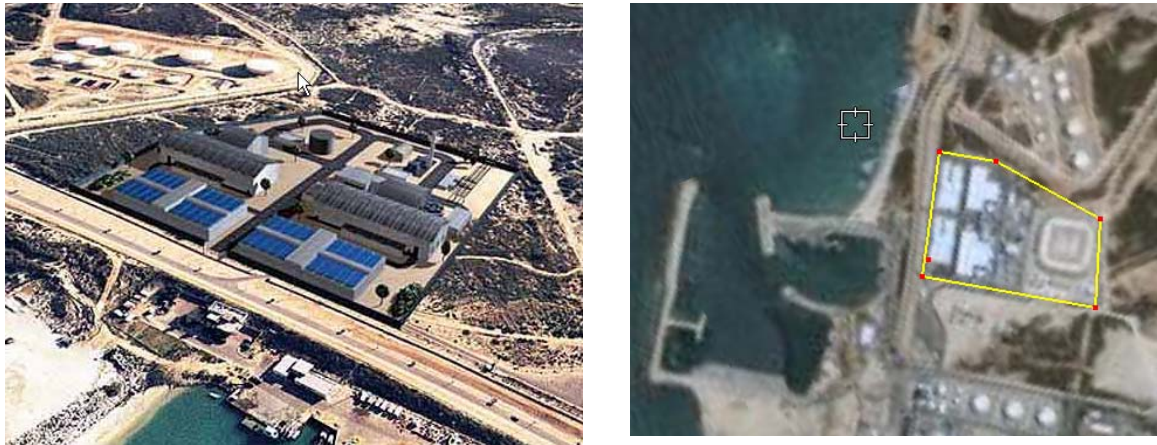
Figure 17 Model of the Ashkelon station and Google Earth R image of the construction site.
