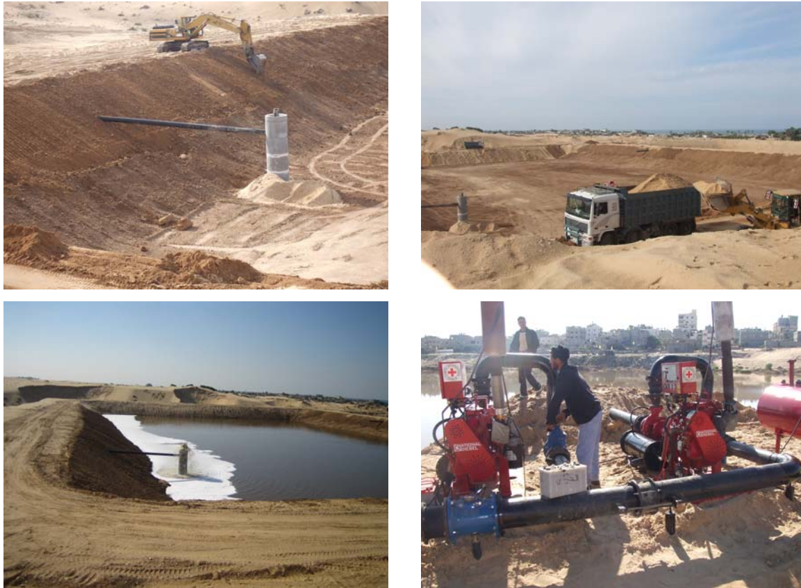
Figure 19 Excavation of the 2 ponds, installation of the pumps and first filling-up of the lagoons at Khan Younis WWTP (Courtesy of the ICRC and Qatar Red Crescent society).
