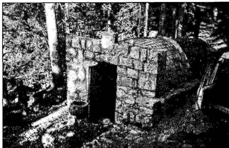
Figure 4: Rehabilitation of a break-pressure chamber.
