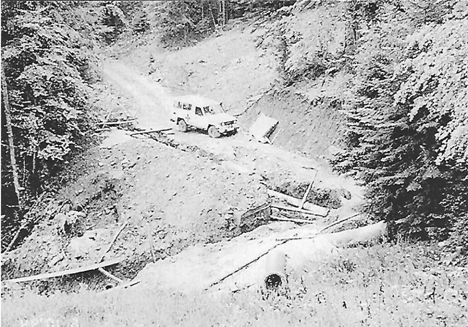
▲ Pale/Sarajevo: Jahorina-Bristica- Brus gravity water supply scheme — repair of leakages in the pipeline resulting from earth movements
